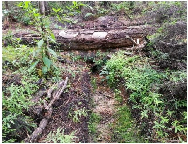
Crossing under the shared path as part of early works
