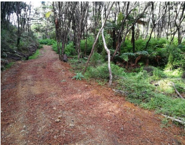
Early works for the construction of the shared paths
