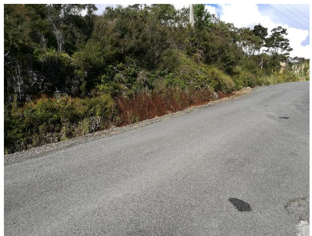
Outlet from the wetland to Thelma Road
