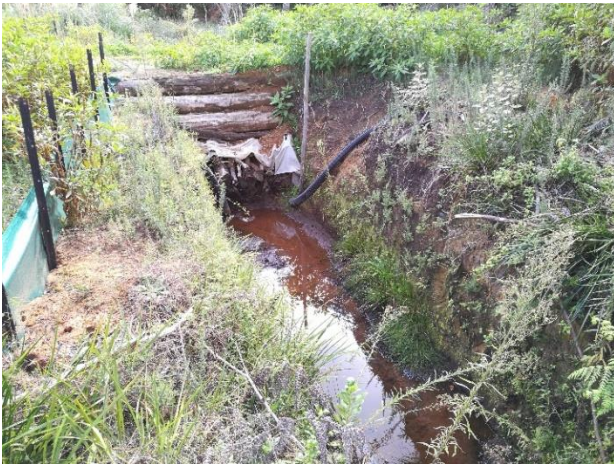
Fascine drain at the outlet from the upstream catchment
