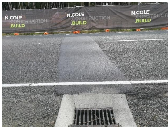
New pipe crossing Molesworth Drive in front of Fire Station development running through the Fire Station development site and discharging to a depression at the rear of the site.
