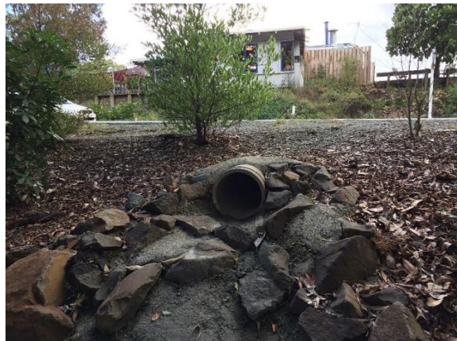
198 Molesworth Drive outlet to existing hollow area
